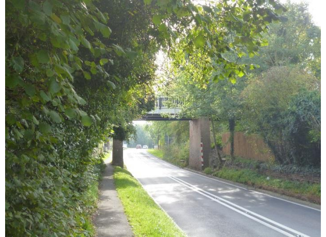
Canal Aqueduct & Walls along A3400
