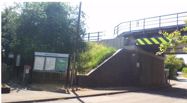
Access to the Station
